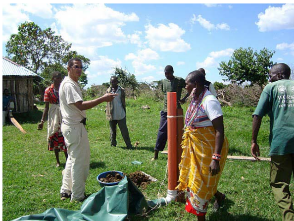
DOMINIC WANJHIA INSTALLING BIO GAS DIGESTER
