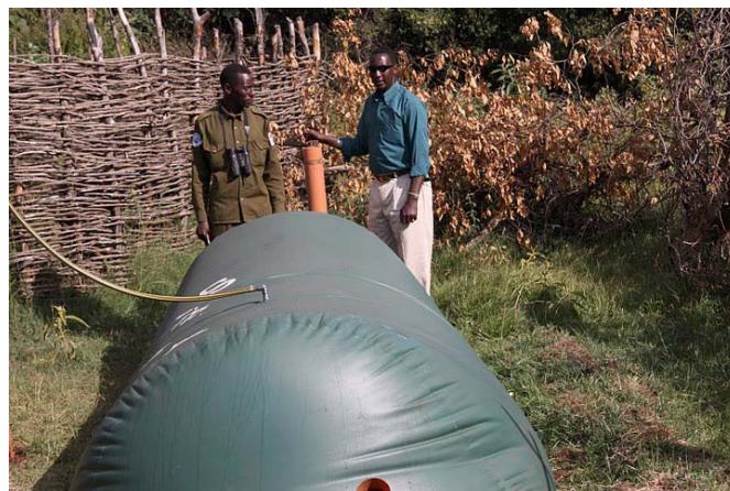
ELIAS & FELIX EXAMINING A BIO GAS DIGESTER
