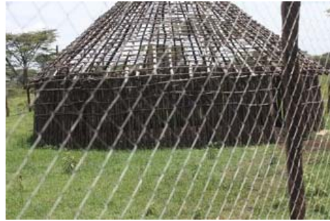
Uncompleted Livestock Enclosure Fortified with Wire
