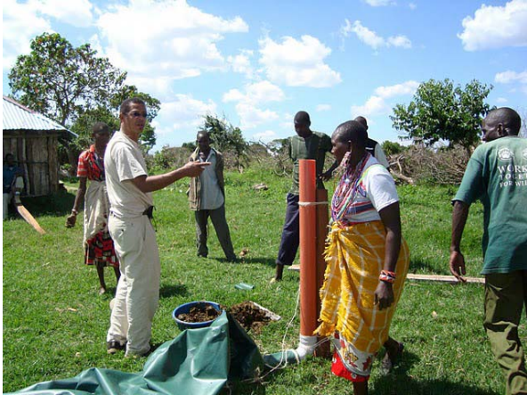
DOMINIC WANJIHIA INSTALLING BIO GAS DIGESTER
