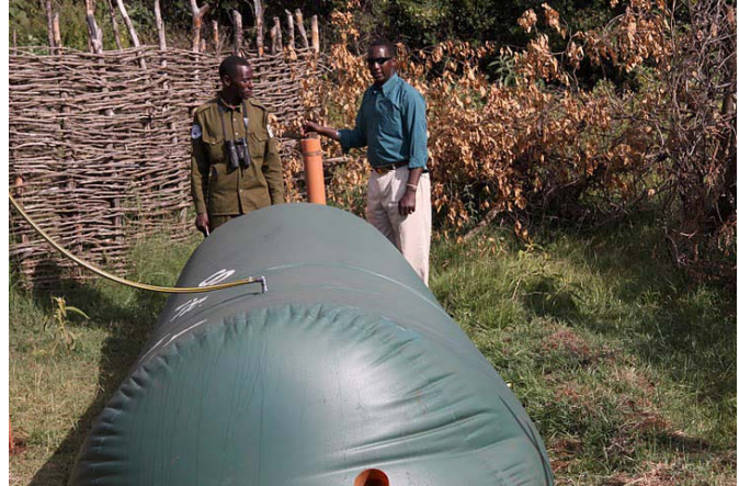
ELIAS & FELIX EXAMINING A BIO GAS DIGESTER
